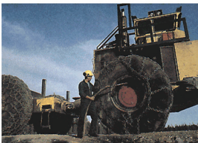
Figure 7. Equipment maintenance (refueling, lubricating, washing, etc.) should be undertaken on stable soil away from riparian areas. The greater the distance from the watercourse, the more opportunity harmful substances have to break down.
